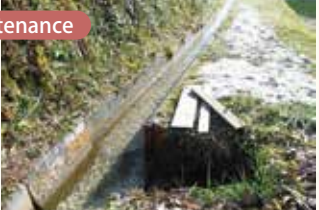
Mizu-otoshi , drainage facilities that prevent the collapse of waterways
